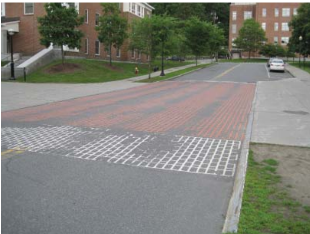
Speed table crossing on Maynard Street. This crossing could be augmented with white bars for greater visibility.
