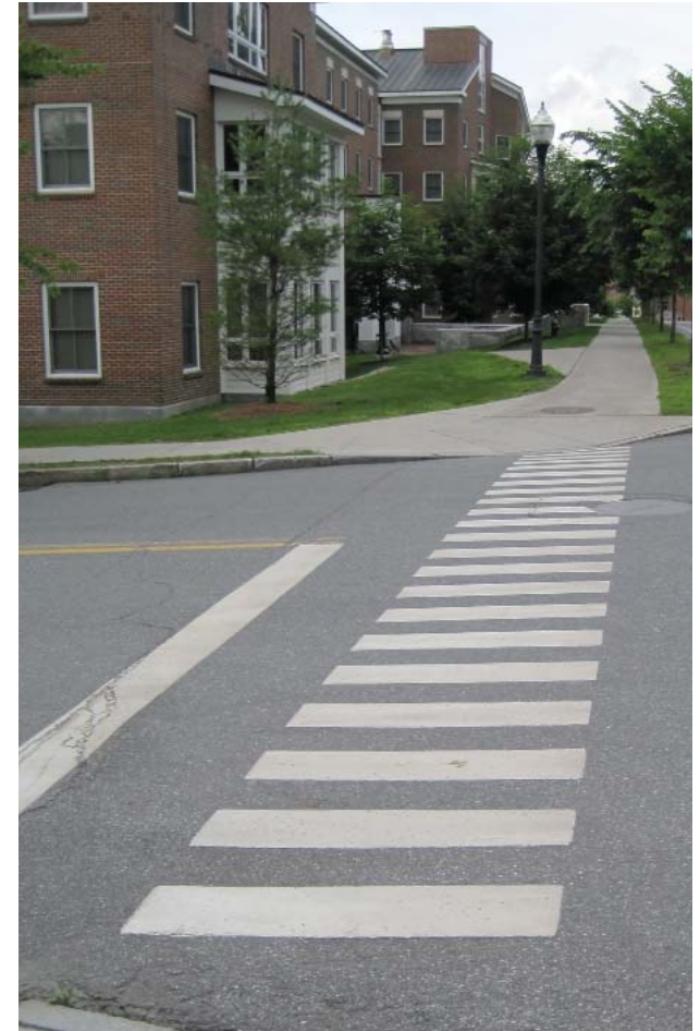
White ladder style crossings.
