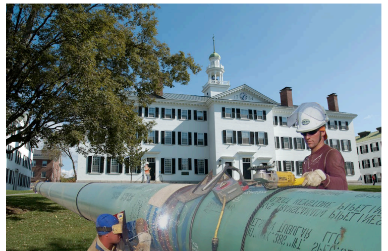
Construction on the Keystone Pipeline has gone a little wonky.
